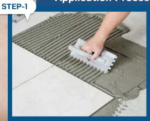
The tile adhesive is applied in a thin layer by means of a notched trowel.
